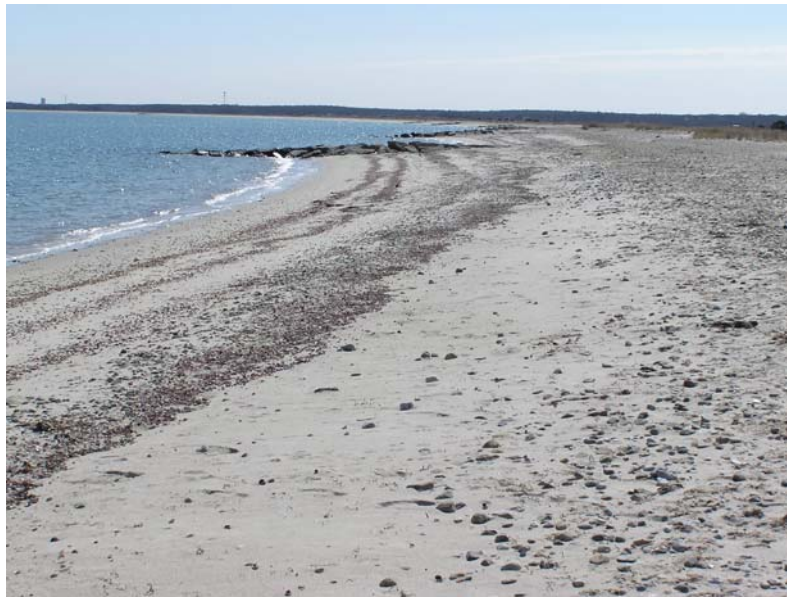
Figure 8. Photograph of stone groins installed south of Little Bridge in 1954.
